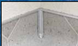
COMPLETE INSIDE CORNER
