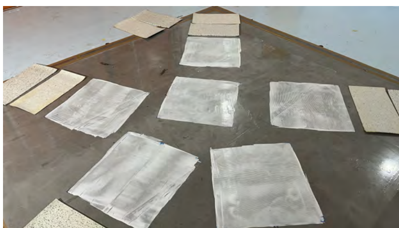
Figure 2.5: Giltgrip 66 adhesive curing
