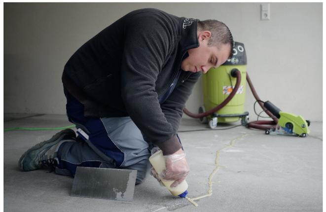
Following the cutting, vacuuming and insertion of the corrugated links, UZIN KR 516 is precisely applied into the joint.
