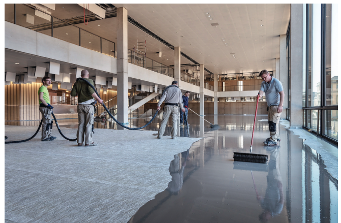
Pump UZIN NC 160 levelling compound over the UZIN RR 201.
