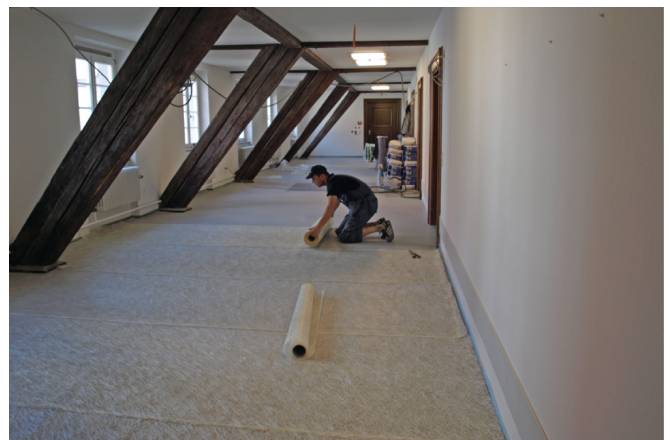
Lay UZIN RR 201 over the entire surface to be renovated.
