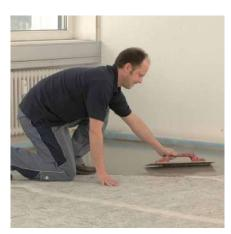
Application of the thin screed UZIN NC 170 + 50 % silica sand 0.3 – 0.8 mm
