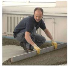
Application of the light weight screed UZIN NC 194 Turbo
