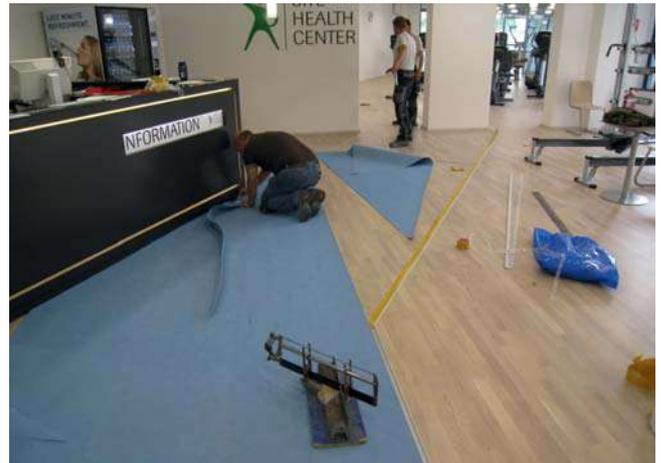
This is a typical situation easy to master with UZIN KE 2000 S NEW: Installation of PVC floor covering during ongoing operation on an installation underlay, here, for example, on UZIN RR 186.
